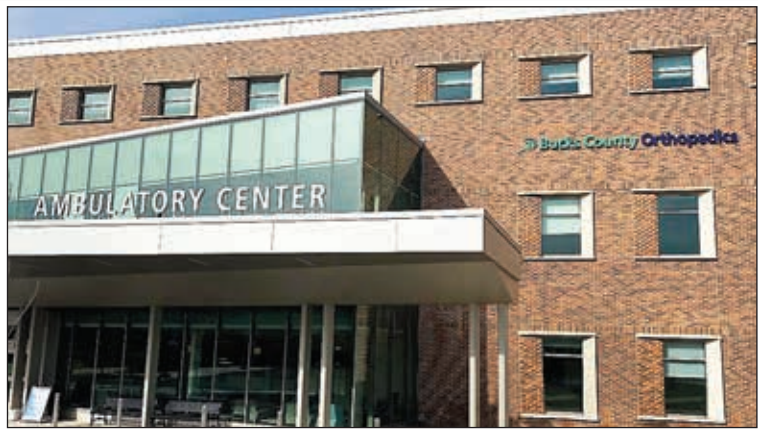
Bucks County Orthopedic Specialists' (BCOS) new office – its third – is located on the main campus of Doylestown Hospital.
